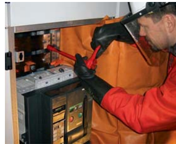
Maintenance of a switchgear system
